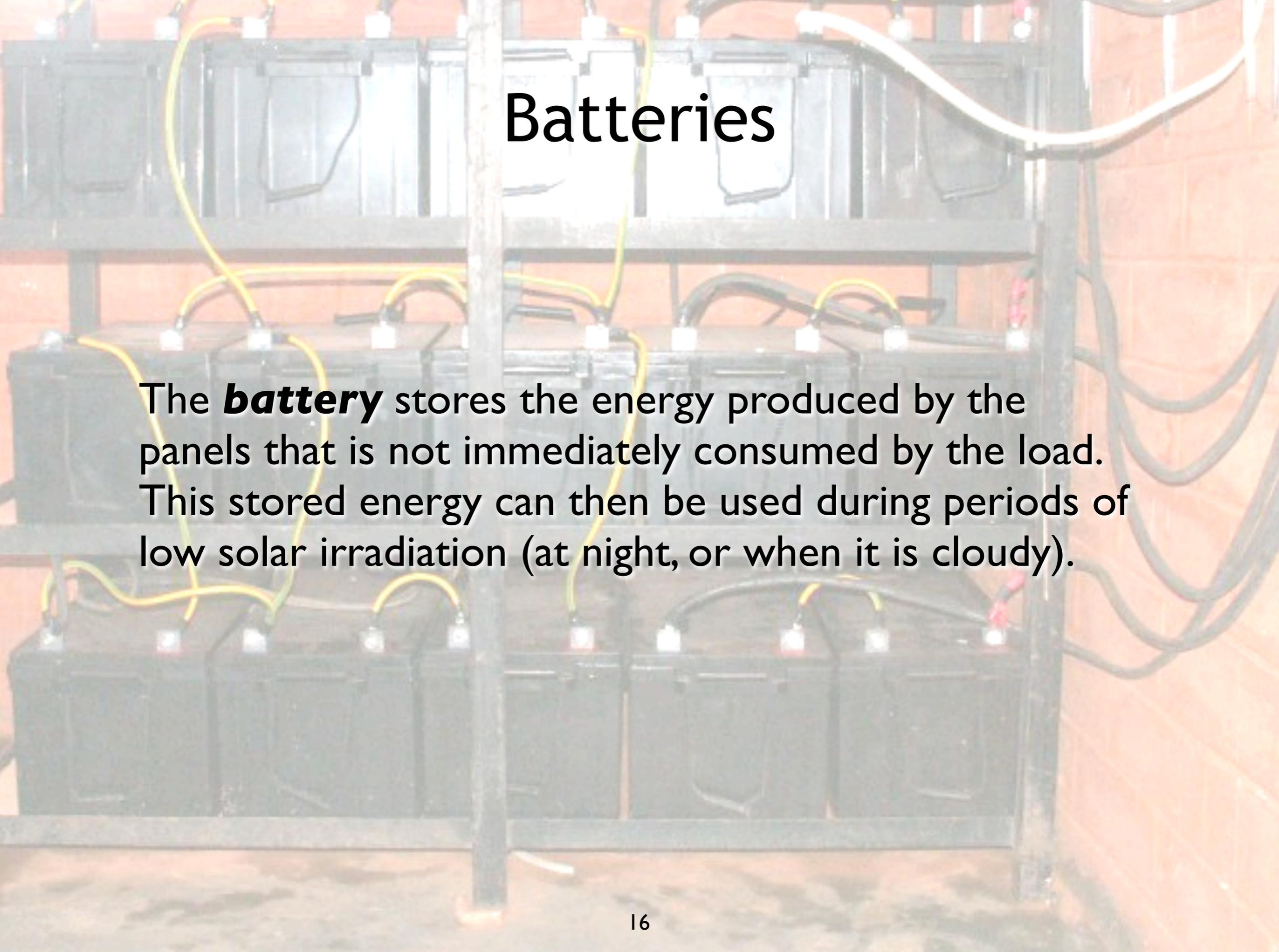
The ***battery*** stores the energy produced by the panels that is not immediately consumed by the load. This stored energy can then be used during periods of low solar irradiation (at night, or when it is cloudy).
