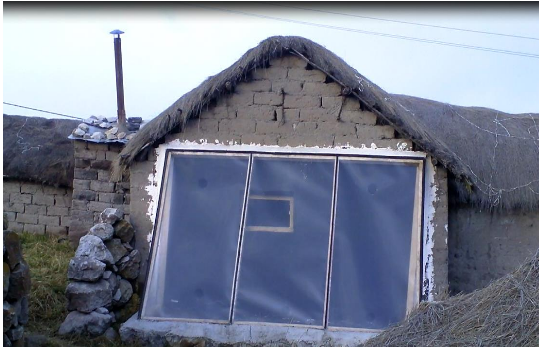
Hot house's technique called "Hot Wall".
