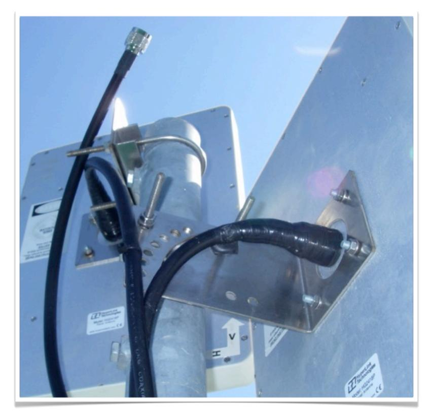
Most antenna problems are caused by coaxial cable connections that loosen due to vibration, allowing moisture to penetrate the connector interface.
