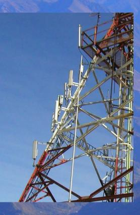
Sectorial Antennas are less affected by the tower and can easily be downtilted. This is particularly necessary when the subscriber is close to the base station or when the base station is much higher. Mechanical downtilting can compensate for the effect of the structure.
