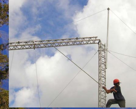
A pulley attached to the top of a pole will facilitate the tower installation
