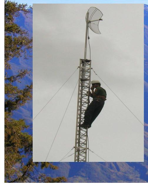
Always use a harness securely attached to the tower when working at heights
