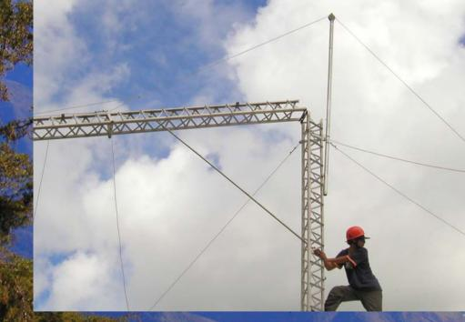
A pulley attached to the top of a pole will facilitate the tower installation
