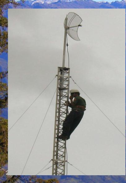
Locate the antennas so that they have clear line of sight to the antennas at the opposite endpoint of the link.
