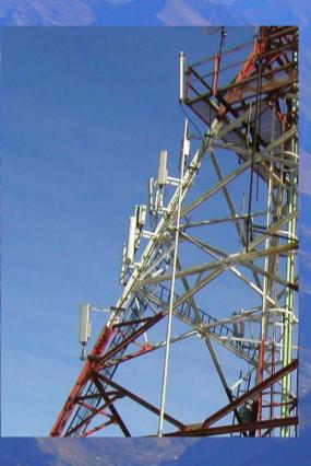
Sectorial Antennas are less affected by the tower and can easily be downtilted. This is particularly necessary when the subscriber is close to the base station or when the base station is much higher. Mechanical downtilting can compensate for the effect of the structure. Electrical downtilting can be accomplished by changing the phase of feeding elements.
