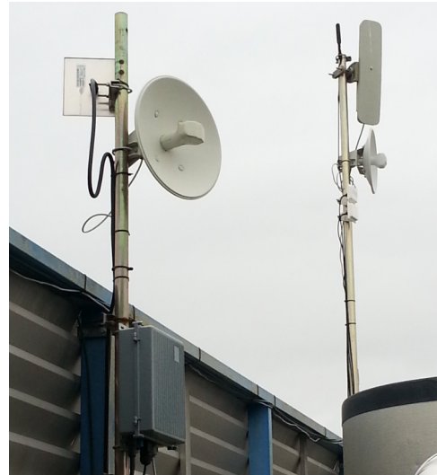
Fig. 2. Super node with outdoor hardware for wireless links between community nodes
