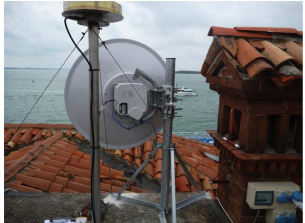
Figure 8: 17 GHz ODU with the integrated antenna.
