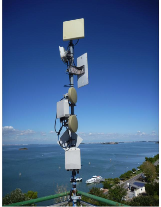
Figure 1: WiMAX base station antennas and point to point links in the roof of San Camillo.
